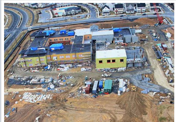
Wilson Wims Elementary School under construction.
